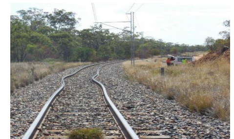
Lateral buckling of the track due to high temperatures
